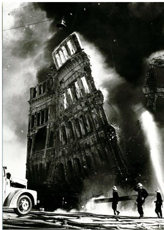
The wall of Buckingham's department store collapses during the fire in Oxford Street on Anzac Day 1968.
