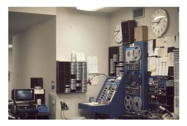
At the bottom of each hour, we fed audio reports and actualities to the stations, playing the segments listed in the hourly billboard that had been recorded onto individual cartridges, or "carts." The large blue machine was a piece of homemade automation equipment that played the carts, and it was affectionately called "pinball." It was called other colorful names when it didn't work right, which was quite often.
