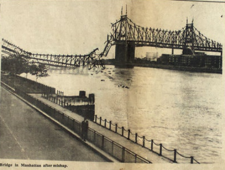
Bridge in Manhattan after mishap.
